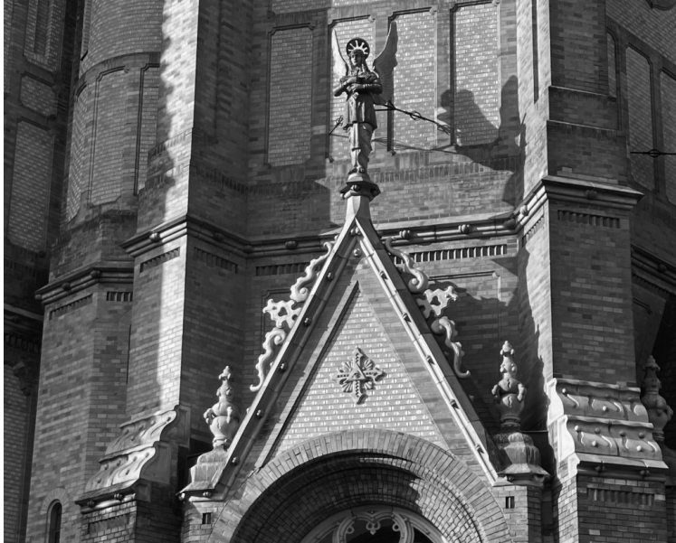
Ill. 1. Church of St. Ladislaus in Budapest – detail of the wimperg with the sculpture of an angel, crockets, pinnacles, and the roof tiles of the buttress bending into Art Nouveau forms (photo by author, 2024)
