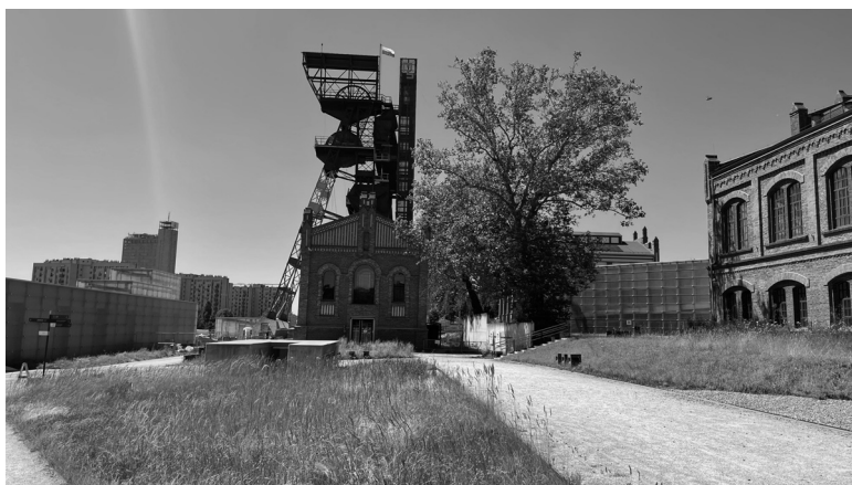
Ill. 4. Silesian Museum in Katowice, revitalized winding tower of the “Warszawa II” shaft – currently a viewing tower, photo by Monika Sroka-Bizoń
