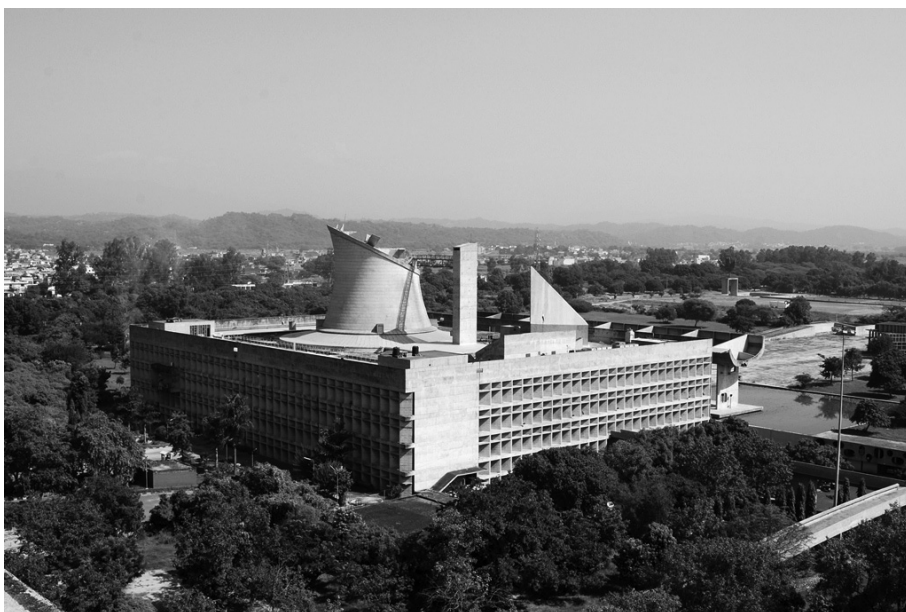
Ill. 1. Palace of the Assembly, Chandigarh, project: Le Corbusier, photo: Sanyam Bahga [in:] Wikimedia Commons, 1.07.2006, https://upload.wikimedia.org/wikipedia/commons/8/86/Assembly_09.jpg (access: 15.09.2025)
