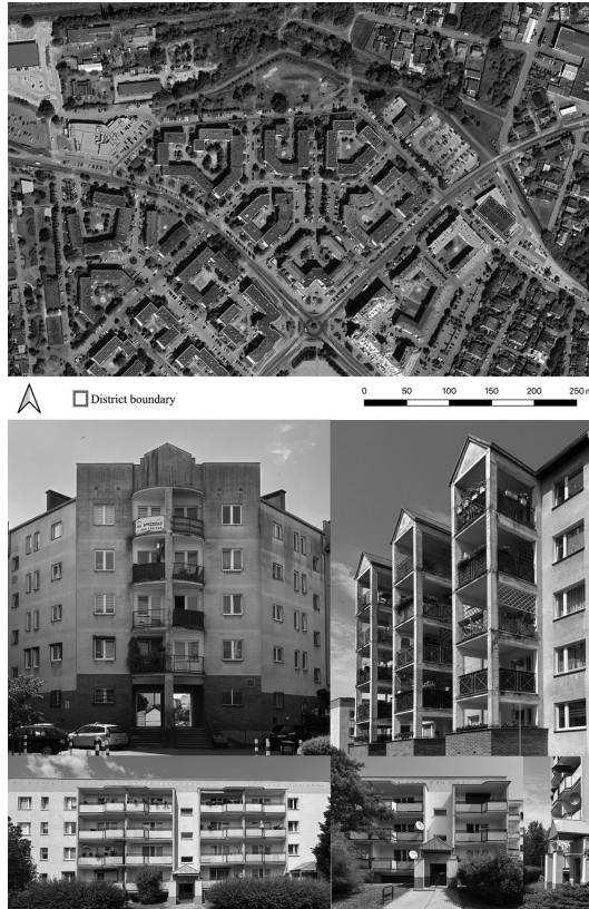
Ill. 3. Cegielskiego estate in Swarzędz. Satellite image downloaded through Google Earth Engine plugin (version 0.0.7) in QGIS 3.40. Collage of photos from on-site visit on 03.07.2025. Own work
