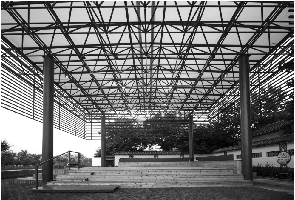
III. 2. A drama stage for the Beihedong Village in Zibo City, Shandong Province, China (by Fu Yingbin). The huge floating skyhook ceiling is applied in the renovation project of rural performance stage, which is provided places for various public activities following the traditional Chinese culture.
