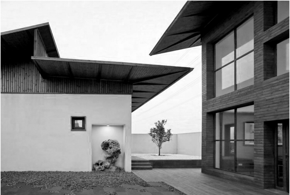
Ill. 4. Deep 3 Courtyard south of Yangtze River, Jiangsu China. The Project is designed by SU Architects (Photo by Shengliang Su) 2015. The project reflects the modern construction technology and living comfort, satisfying the spiritual needs for those Chinese who still really treasured Chinese traditional Cultures of living themselves to the nature.
