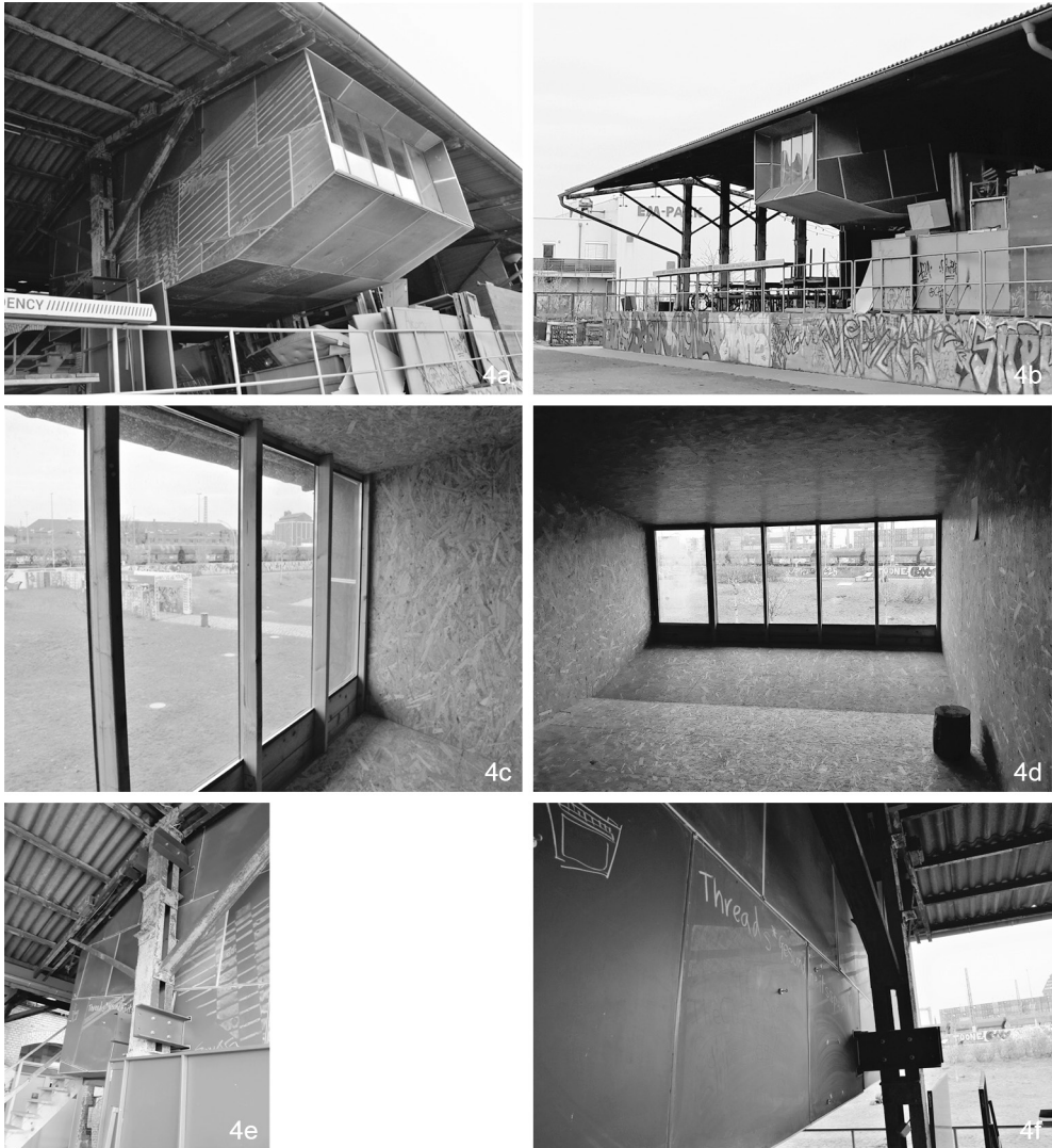
II. 4. Center of Art and Urban Planning (ZK / U), Berlin. Research on the possibilities of developing structures complementing the basic form, based on solutions and non-obvious materials. Author's photo; a) and b) a workshop pavilion suspended above the terrace located at the back of the building, in the immediate vicinity of the social garden established on the rest of the area; c) and d) the transparent wall of the pavilion crops openly to the social urban garden and further to the surrounding industrial buildings; e) and f) for the needs of the new structure, the cover of which was made of old school boards, the roof terrace roof support structure was used. Part of the pavilion's construction comes from recycled materials
