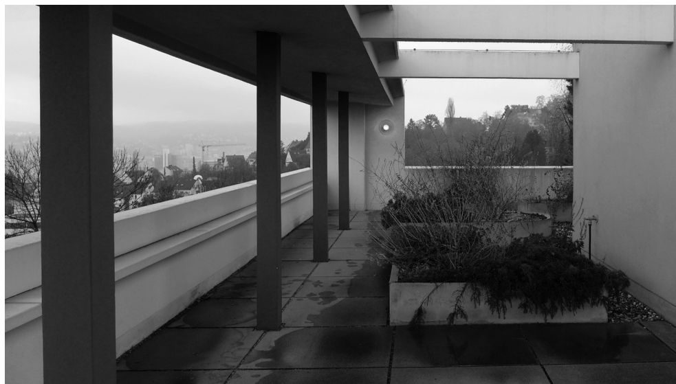
III. 4. Terrace on the uppermost storey of the semi-detached house on the Weissenhof estate in Stuttgart. The roof that frames views of the landscape and greenery that is present on the roof of the building provides its residents with contact with nature. Original photograph
