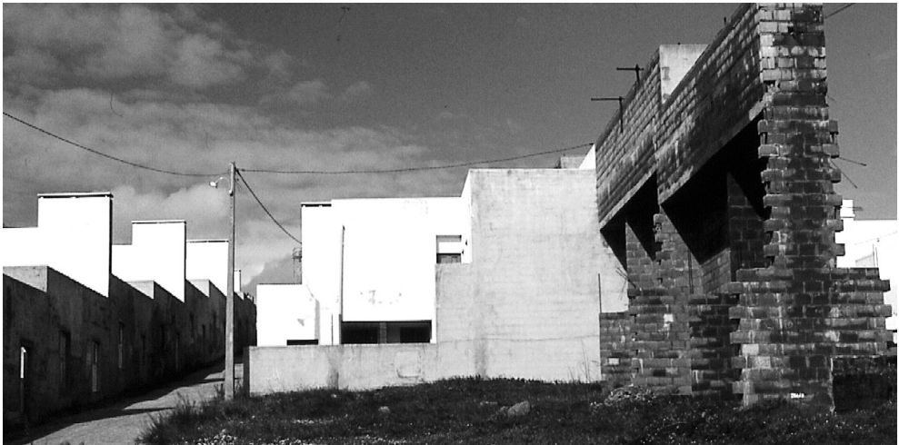
Ill. 2. A. Siza, Social housing in Quinta da Malageira, Evora, photo by the author
