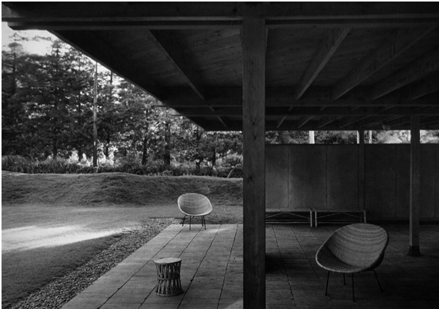
Ill. 4. View of ground floor, source: ArchEyes Team, Seijo Villa: Kenzo Tange's residential masterpiece [in:] ArchEyes, 21.02.2023, https://archeyes.com/kenzo-tanges-house-villa-seijo/ (access: 12.09.2025)
