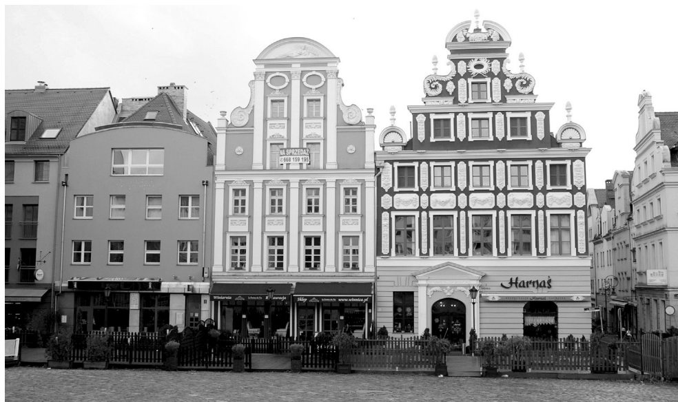
Ill. 4. Szczecin – Old Town, Sienna Market, reconstruction of baroque facades from the 17th century (original red and blue colors). Author's photography 2017
