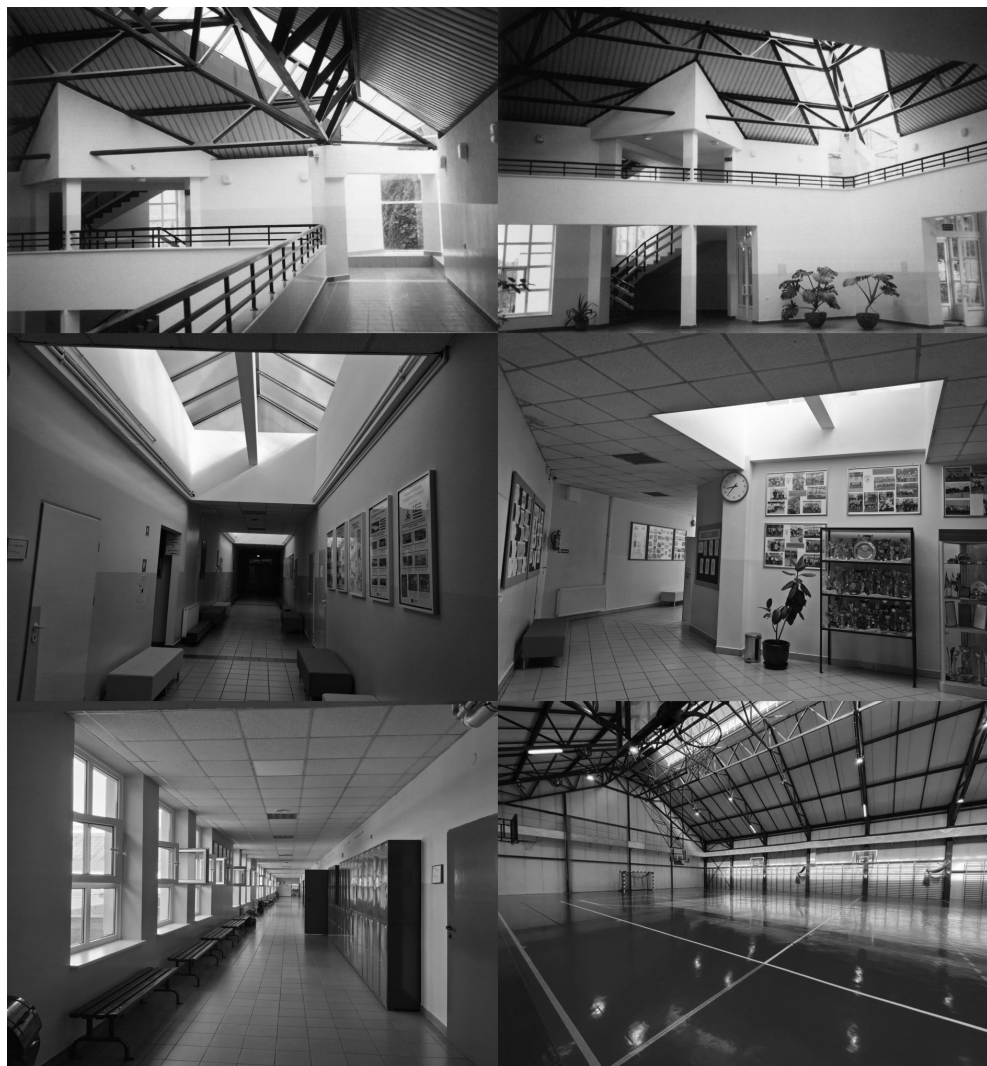
III. 4. Holy Father John Paul II School Complex in Niepołomice, ul. Kazimierza Wielkiego 1 in Niepołomice, Chief Designer and Author – architect Mieczysław Gała, authorship collaboration: architect Ewa Kasz, architect Marta Kozielec, collaboration on the second version of the sports sector: architect Miłosz Łucki. Phased implementation 1994–1999. Photos: architect Mieczysław Gała gallery and interior of the school forum, architect Monika Gała-Walczowska skylights and internal communication spaces of the school, source of illustrations: Archive of architect Mieczysław Gała and the Monika Gała-Walczowska Architektura Design Studio; interior of the gym, source: Sala Gimnastyczna [in:] Zespół Szkół im. Ojca Świętego Jana Pawła II w Niepołomicach , https://www.lo-niepolomice.pl/a/sala-gimnastyczna-1 (access: 6.09.2025)
