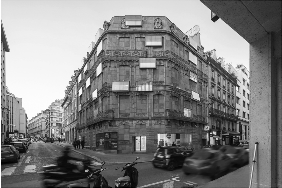
Ill. 8. Hotel Fouquet's Barrière, front facade, source: L. Ghinitoiu, A Complementary Architectural Dialogue of Past and Present in the Refurbishment of Hotel Fouquet Barrière [in:] ArchDaily, https://www.archdaily.com/915677/a-complementary-architectural-dialogue-of-past-and-present-in-the-refurbishment-of-hotel-fouquet-barriere/5cbf18ad284dd19951000051-a-complementary-architectural-dialogue-of-past-and-present-in-the-refurbishment-of-hotel-fouquet-barriere-photo?next_project=no (access: 15.08.2025)
