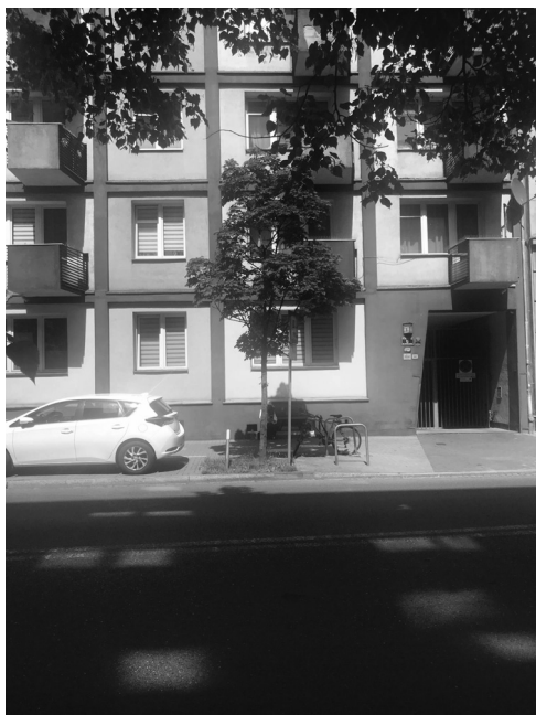
III. 5. The detail of the ground floor at 5 Mazowiecka Street, Krakow, photo: F. Suchoń
