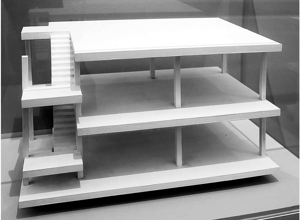
III. 1. Model of Dom-ino system, arch. Le Corbusier, 1914 / source: Wikimedia Creative Commons, CC Gemeentemuseum Den Haag
