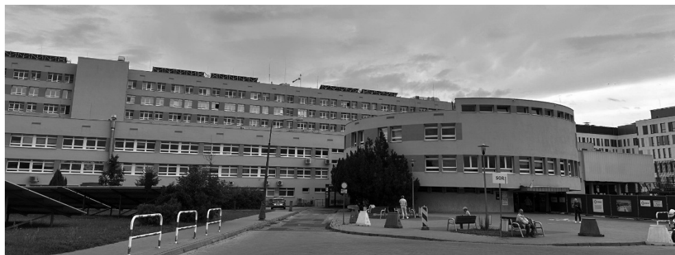
Ill. 2. Provincial Hospital in Poznań, photo by author
