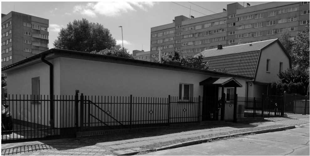
Ill. 2. Kaliny Housing Estate in Szczecin with a single-family housing complex A housing estate of one-storey, repetitive residential houses established in the 1960s (house on the left). Since the beginning of the 1990s it has been undergoing systematic reconstruction – „vernacularization” (house on the right). The architectural form is being fundamentally changed, new roof volumes and decorations are being introduced.
