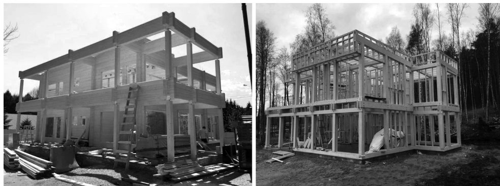
III. 1. Assembly of a building using a prefabricated timber log system – massive wall elements laid in layers (left photo). Timber frame construction during assembly – a lightweight frame consisting of vertical and horizontal members (right photo), source: Technology [in:] EcoHauseMart, https://ecohousemart.com/technology/ (access: 14.07.2025)
