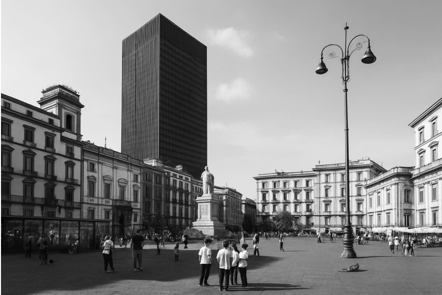
Ill. 5. Seagram Building from Dante Square in Naples . AI composition made by author and Joshua Flenghi, 2025
