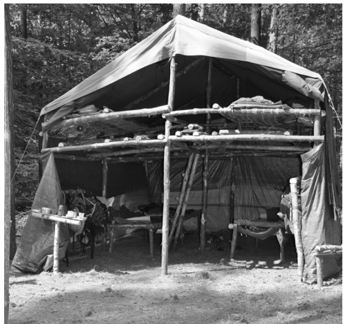
Ill. 13. Two-tier tent, kurnik ('hen house'). By elevating the tent, the builders gained another 20 m 2 of useful floor area. 1 st KDH Trop ('Trail'), Kujanki 12.7.2016, photographed by the author
