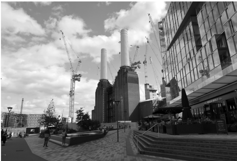
Ill. 5. Battersea Power Station development in 2018. Photo by A. Jozwik 2018
